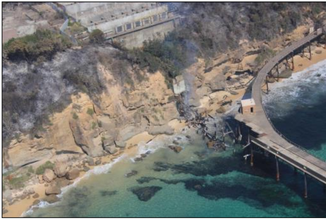
25. Coal from the loading chute in the cliff had been spilt onto the wooden jetty. This was ignited by falling embers during the 2013 fire. (Photo R Miller).
