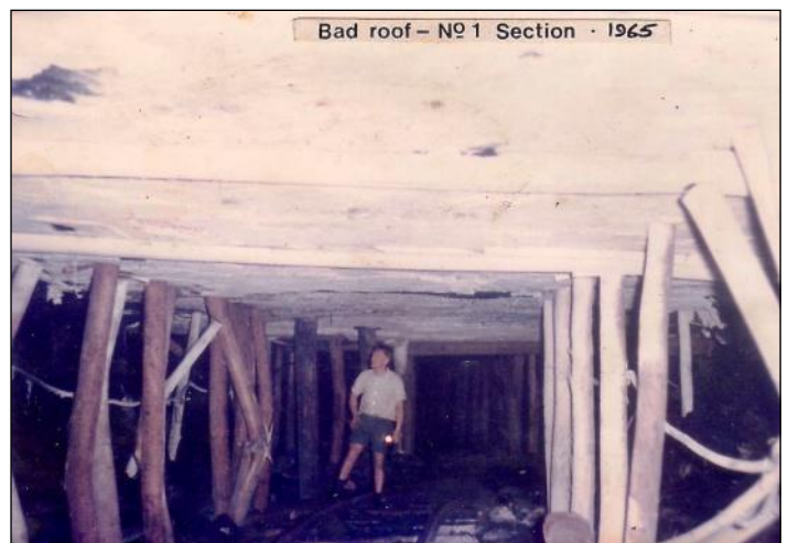
18. Expansion in the claystone roof. (Photo from the ELMHS Collection).
