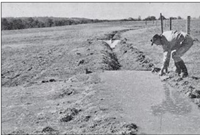
10. Blocking the channels at various points allowed Yeomans to determine which parts of the valley side would be irrigated. (From Yeomans Keyline Farming Explained).
