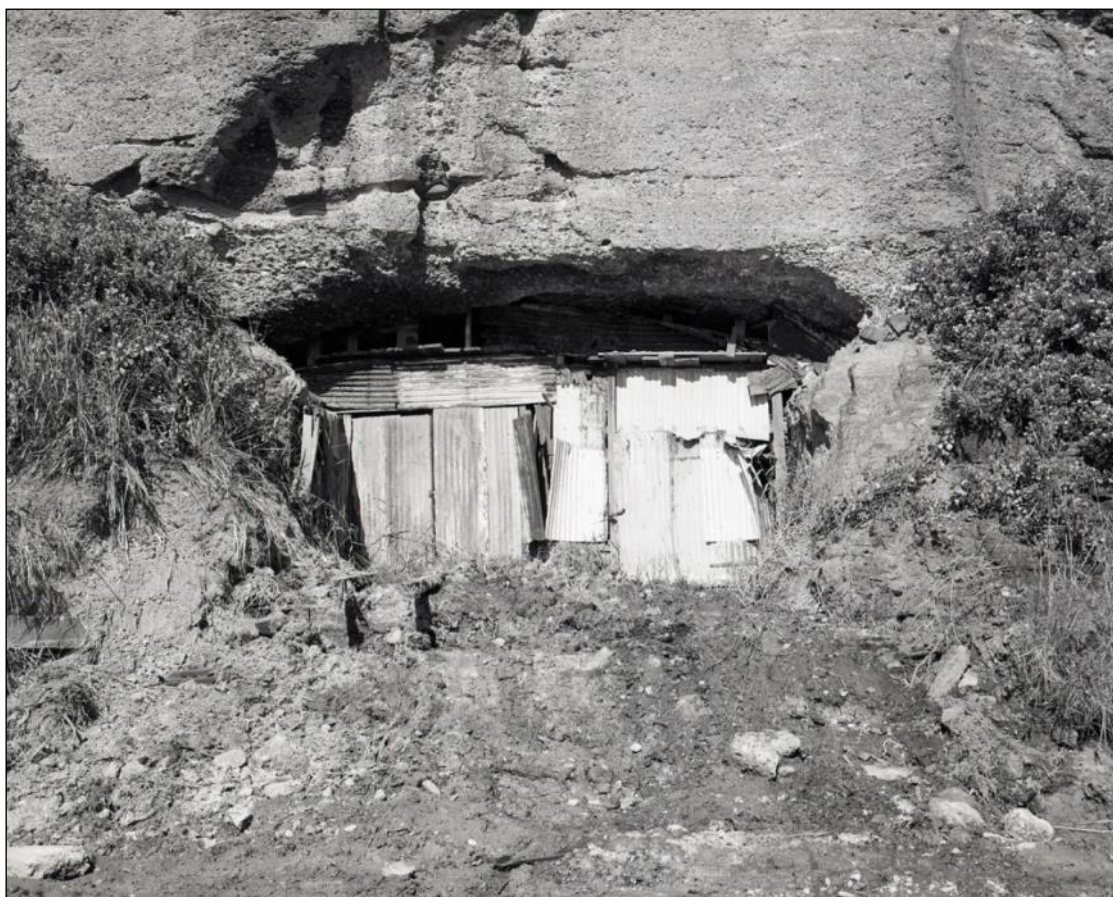
2. The larger shaft remained opened after the colliery closed and at times fishermen used it to store boats. It was sealed with concrete in 2003. (Photo from the ELMHS Collection).
