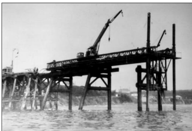
30 & 31. A Bailey bridge was used to repair and rebuild the second jetty. The wooden frames were replaced with steel. (Photos from the ELMHS Collection).
