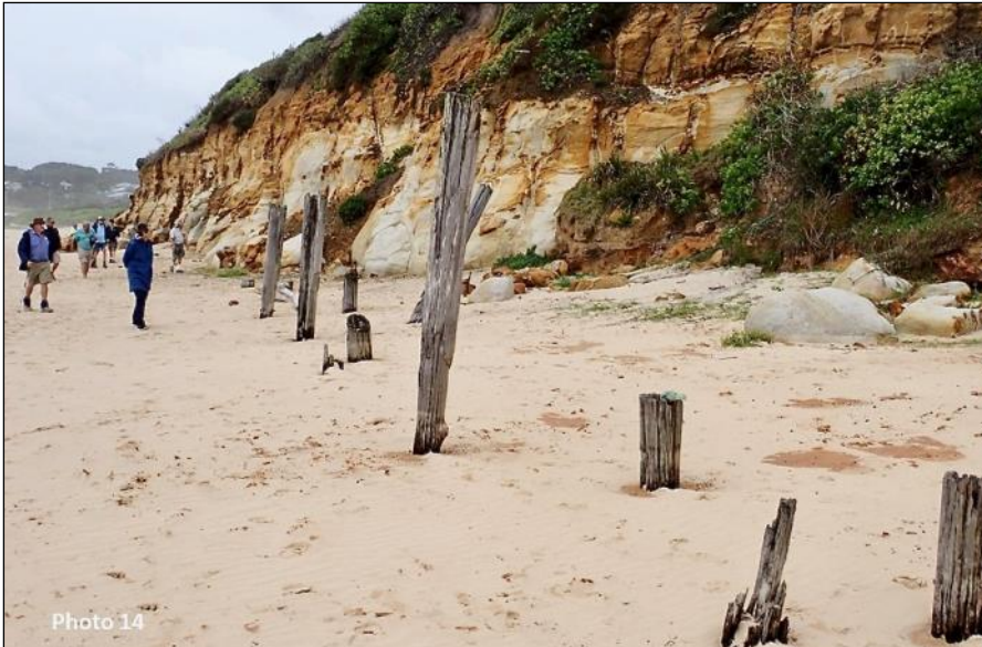
14. Piles from a break wall created to prevent erosion on the coastal railway. (Photo by Chris Morton).
