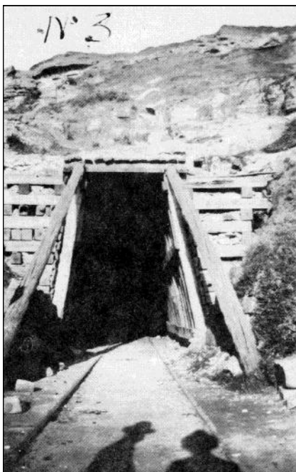
5. Northern exit of No. 1 tunnel. Note the narrow top - the tunnel was designed for horse and dray.
