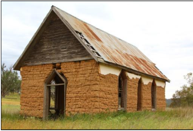
51. An old pisé constructed church showing the horizontal layers of rammed earth and the whitewashed covering render.
