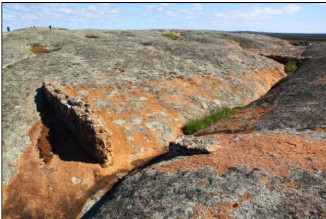
100. Small stone dam walls across rillen.
