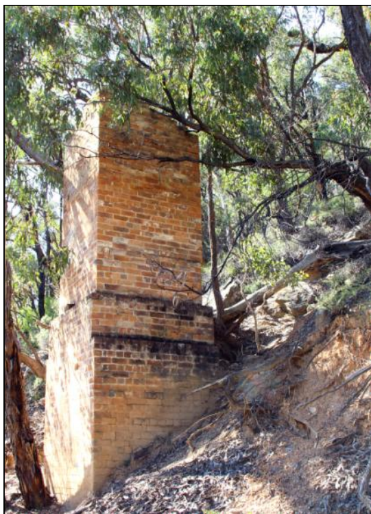
5. Brick ventilation chimney.
