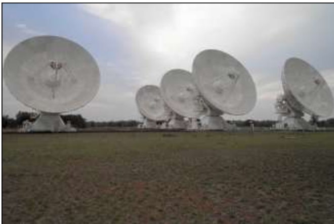
18. The five mobile dishes of the Australia radio telescope. The sixth fixed dish is situated 5km away.
