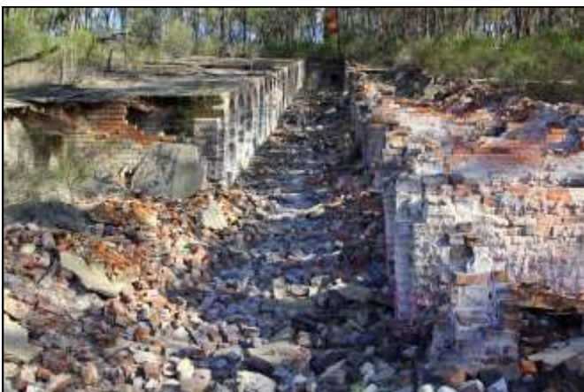
14. Brick arsenic (pink deposits) condensers, Ottery Mine.
